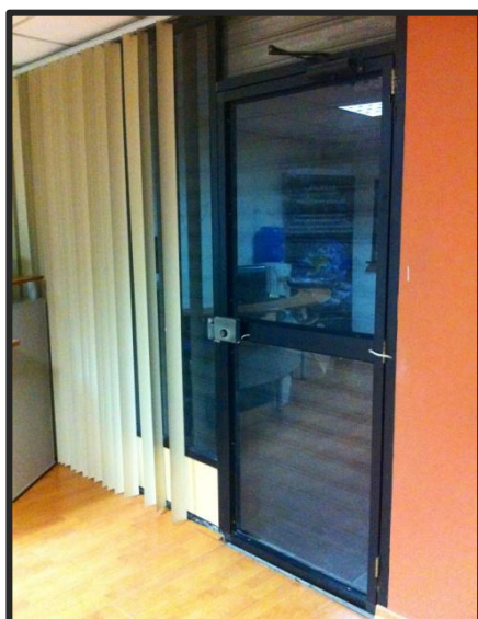
Foto 6: Vista interior puerta principal
