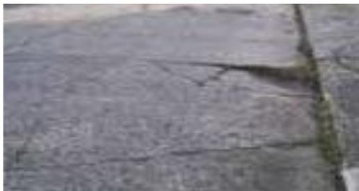
*Figura 14: Levantamiento losa Fuentes: (SCRIBD, 2017)*
